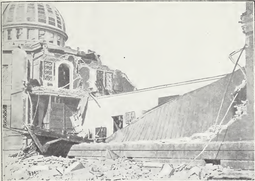
A. COMPARATIVE BEHAVIOR OF REENFORCED CONCRETE AND BRICKWORK UNDER EARTHQUAKE VIBRATION, MUSEUM, LELAND STANFORD JUNIOR UNIVERSITY.
